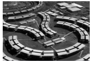
NON-PROCESS INFRASTRUCTURE Koodaideri Stage 3 & 4, WA
