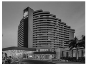
COMMERCIAL FIT OUT Star Casino, NSW
